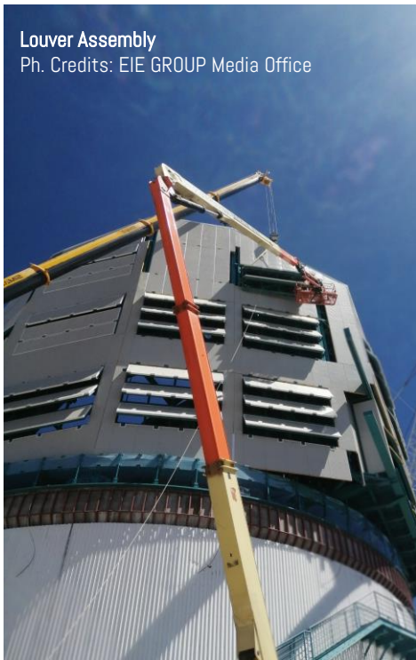
Cladding Installation phase Ph. Credits: EIE GROUP Media Office
